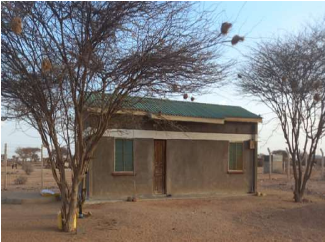
Situation Before Intervention
