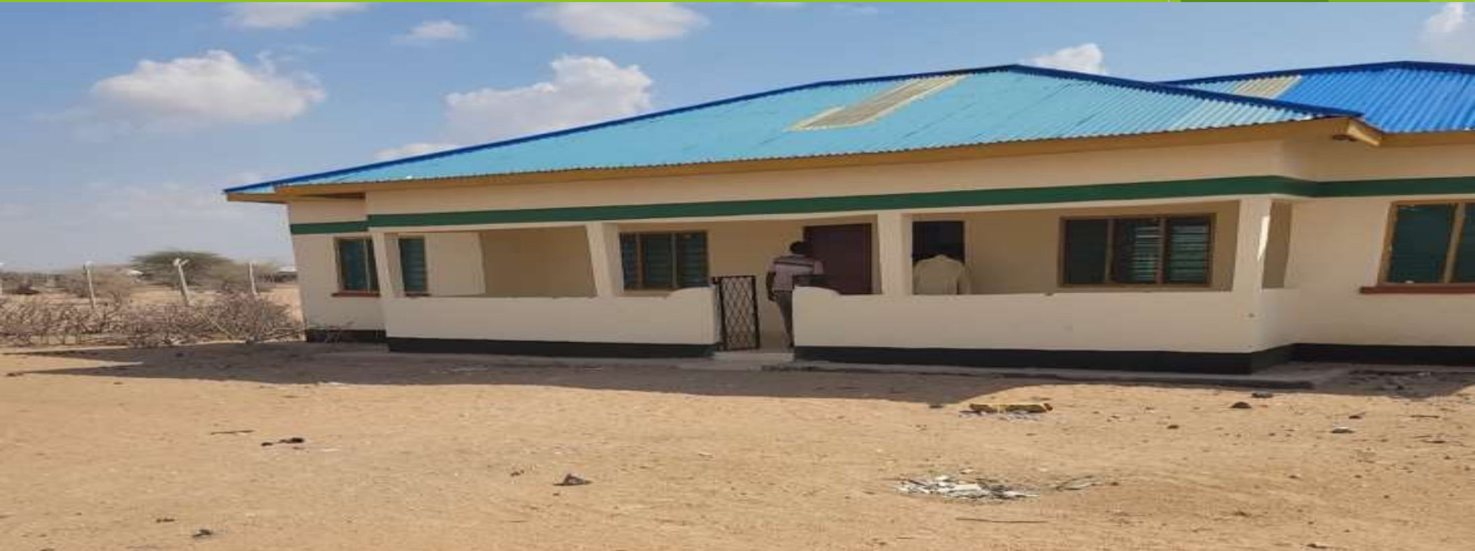
Construction of staff quarters Shanta Abak , Garissa
